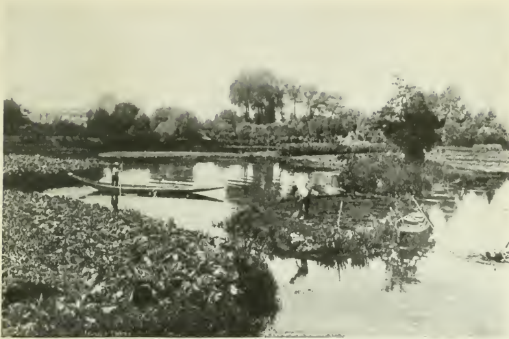
THE "HORTILLONNAGES" (KITCHEN GARDENS)
